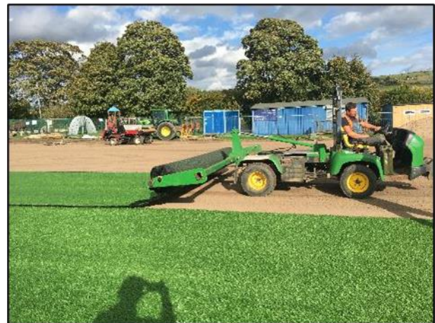
Figure 3. Hybrid carpet installation at Siddal.
