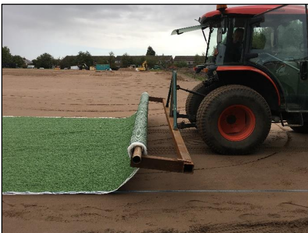
Figure 2. Hybrid carpet installation at Thatto.
