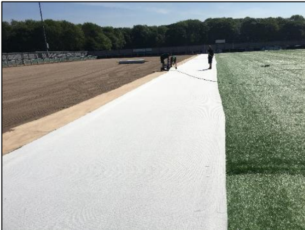
Figure 3. Hybrid carpet installation at Runcorn Linnets.
