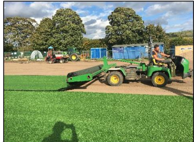
Figure 4. Hybrid carpet installation at Siddal.
